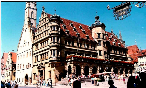
Figure 17-52 The Rathaus or town hall in Rothenburg. This is a beautiful example of unusual medieval architecture.
