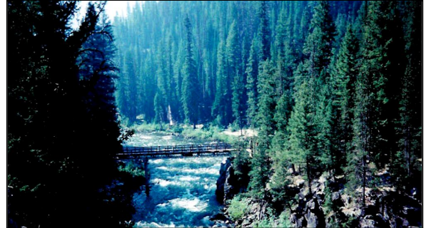
Figure 18-148 New stock bridge in 1999. Our camp was just to the right in the trees.
