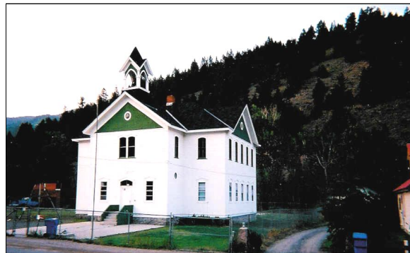
Figure 18-182 An old school directly across the street from the cottage and still in use.
