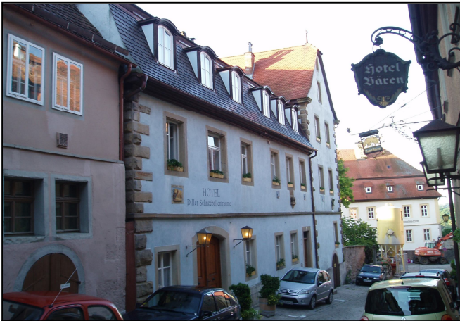
Figure 19-66 The front and main entrance to the hotel Garni-Diller or Diller Schneeballentraum.
