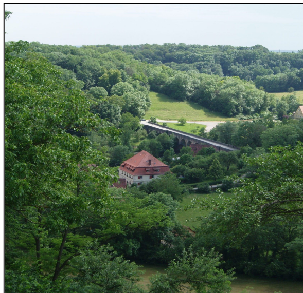
Figure 19-79 A view of the Tauber River bridge, as taken from the wall, I believe.
