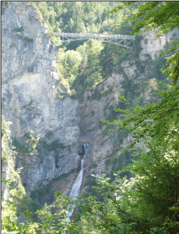
Figure 19-171 The Marienbrücke Bridge as seen from a castle window.
