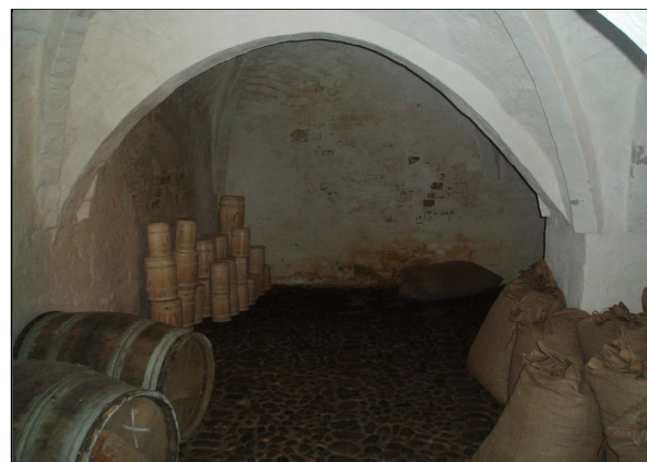
Figure 19-189 A storage area of the old castle similar to those of Von Niepberg.
