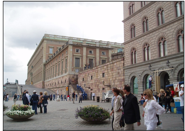
Figure 19-214 The Swedish castle in active use as seen from the plaza in front of it.
