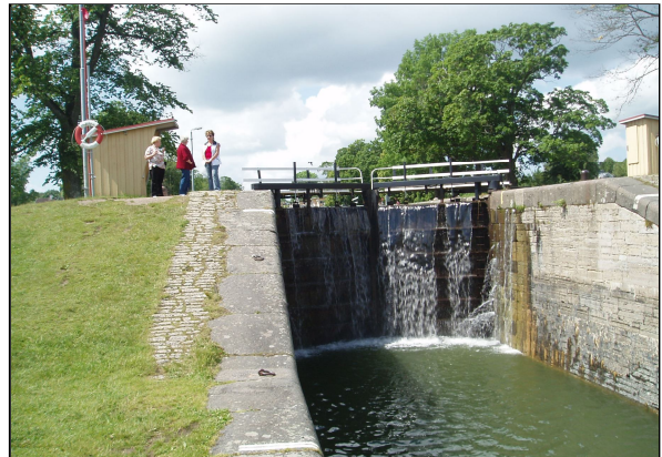
Figure 19-210 A lock on the Gota Canal that has been filled to raise a boat one level.
