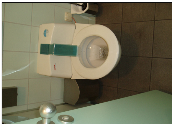
Figure 19-182 A cutting edge toilet seat design that scrubs the seat after each use.
