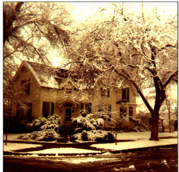
Figure 2-28 A winter scene of the Artie Obenchain home on 17 th and Irene Streets.
