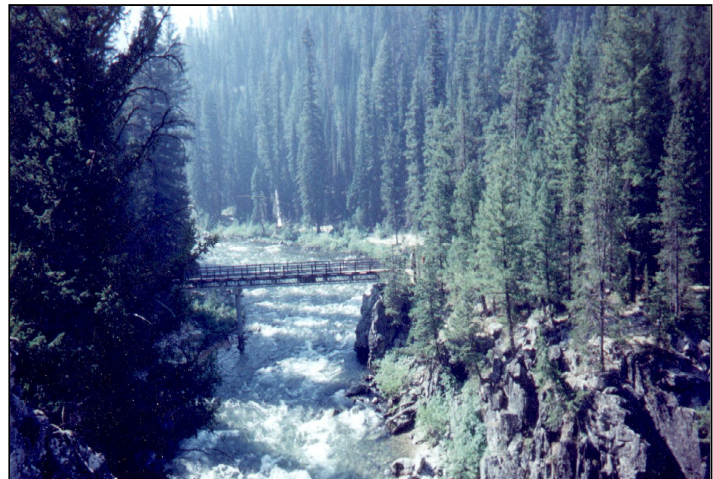
Figure 3-47 The new stock bridge crossing the Middle Fork of the Salmon River in 1999.
