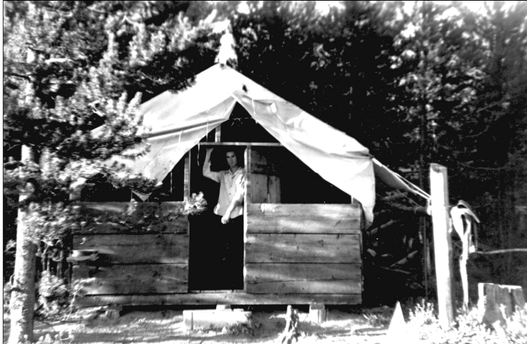
Figure 3-37 "Yours Truly" in the doorway of our humble home located behind the Elk Creek Ranger Station.
