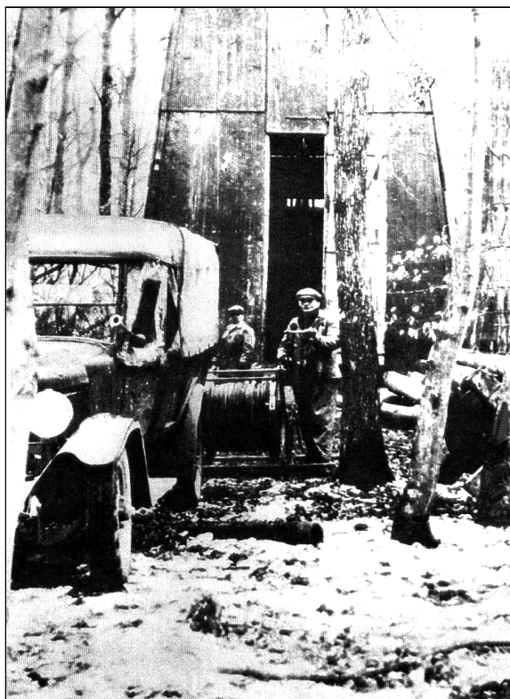
Figure 6-2 Logging a well in Pechelbronn, France in the 1920s.
