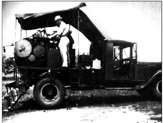
Figure 6-3 William Gillingham & a Schlumberger truck logging a well near Houston, Texas in 1934.
